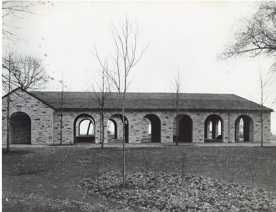
Photo 17: Iowa Building west façade looking east, 1936, Chicago Park District Records: Photographs, Special Collections, Chicago Public Library
