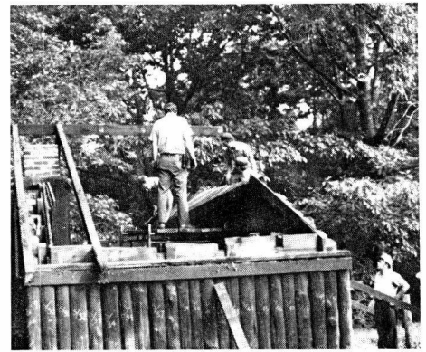
Workers from the staffs of Independence and Valley Forge NHPs carefully disassemble the log cabin.
