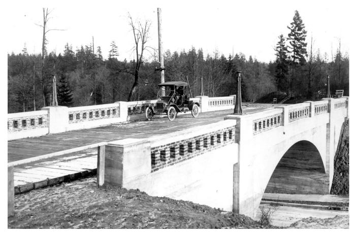
encounter a narrow bridge. According to Don Sherwood, this concrete bridge was built in 1912 to replace an earlier structure with low clearance. As the gully running underneath became increasingly used by cars, a bridge with clearance "ample for modern trucks and moving vans" was required.
