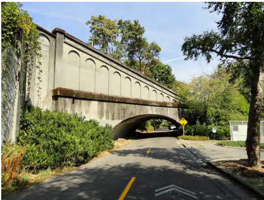
Photo 10. WA_KingCounty_LakeWashingtonBoulevard_0010. Lake Washington Boulevard passes at the Yesler Way trestle bridge (NRHP-listed city landmark), view northeast.
