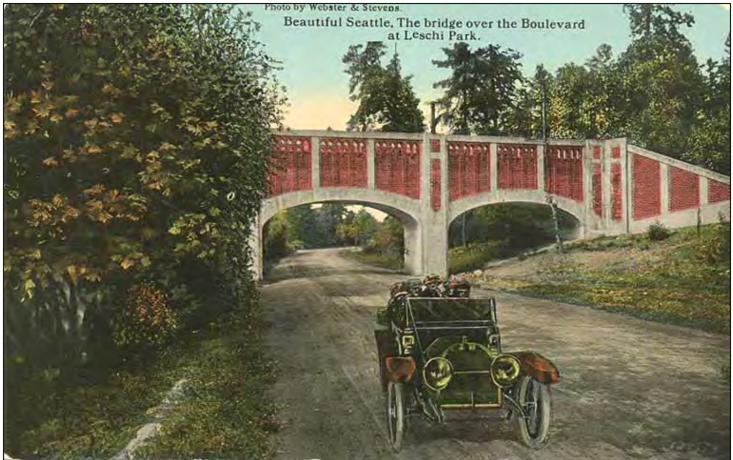
Figure 6. Postcard of "the bridge over the Boulevard at Leschi Park." The postcard is mislabeled, as this is the aqueduct in present-day Washington Park Arboretum as it crosses over Lake Washington Boulevard. Photographer: Webster & Stevens. Image SEA2008, UW28189z. Courtesy of the Seattle Photograph Collection via the University of Washington Library Digital Collections.
