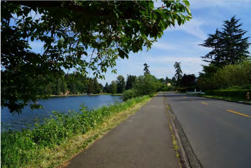
Photo 24. WA_KingCounty_LakeWashingtonBoulevard_0024. Lake Washington Boulevard approaching Seward Park, view south.
