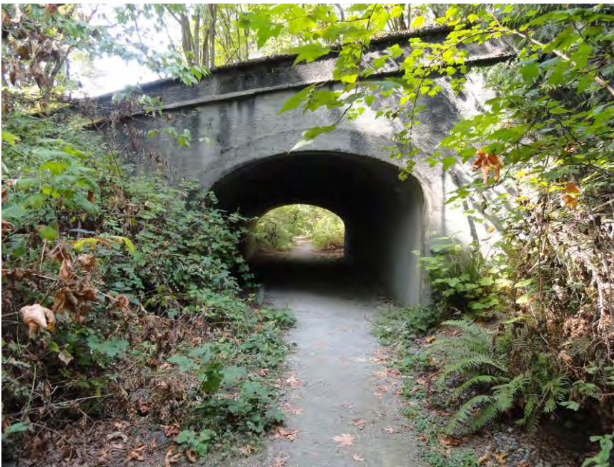
Photo 17. WA_KingCounty_LakeWashingtonBoulevard_0017. Colman Park Overpass No. 2, view north.
