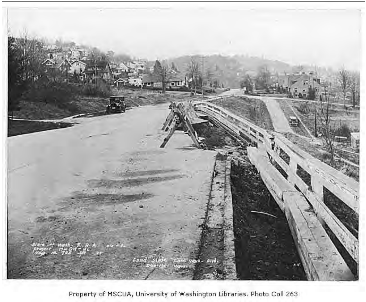
Figure 10. Mudslide damage on Lake Washington Boulevard, March 13, 1935, at present-day location of the South Charles Street Bed. Image UW20579z, courtesy of the Federal Emergency Relief Administration Photographs via the University of Washington Library Digital Collection.
