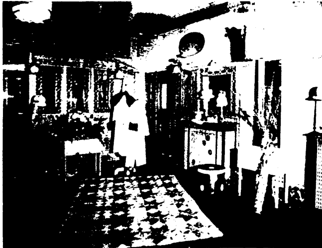
Ca 1940s photograph of a former first floor retail space in the Davenport Hotel. Source: Spokane Public Library.
