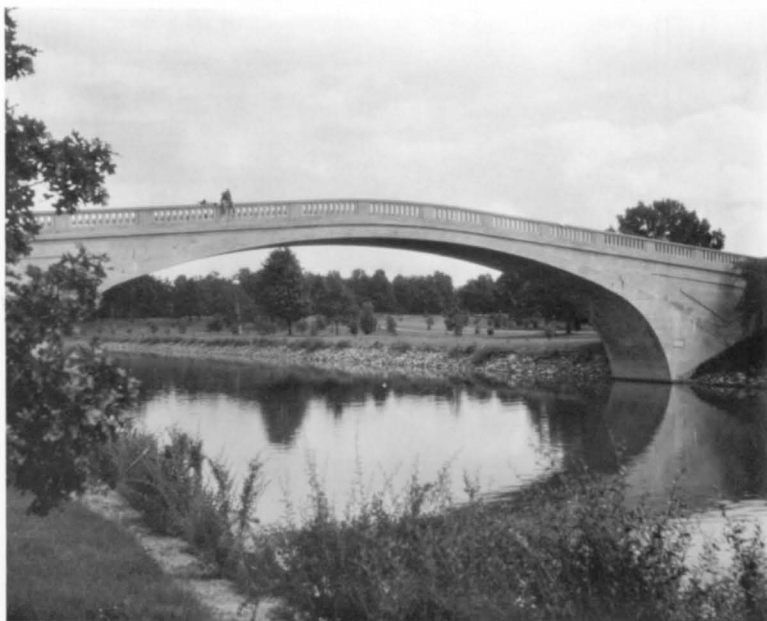
The pedestrian bridge over the New York State Barge Canal at Genesee Valley Park created an unintrusive crossing through the middle of the park as it reflected in the water.
