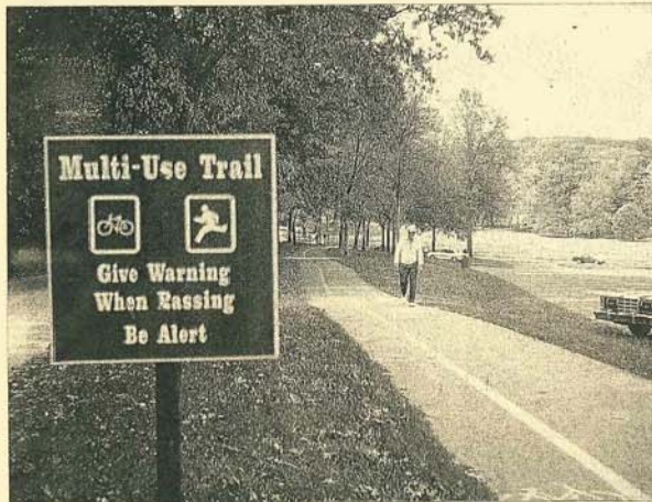
A paved multi-use path at Valley Forge National Historical Park was initially constructed with an 8-foot width, but then became so popular that striping and warning signs had to be installed. (Andropogon Associates, 1993)
