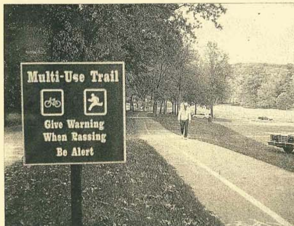
A paved multi-use path at Valley Forge National Historical Park was initially constructed with an 8-foot width, but then became so popular that striping and warning signs had to be installed. (Andropogon Associates, 1993)
