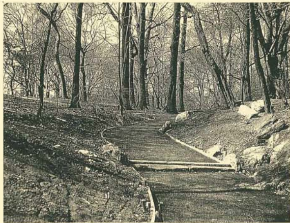
Woodland path restoration in Central Park's North Woods included drainage infrastructure and stabilization of adjacent woodland slopes which had been badly eroded and trampled. (Andropogon Associates, 1993)
