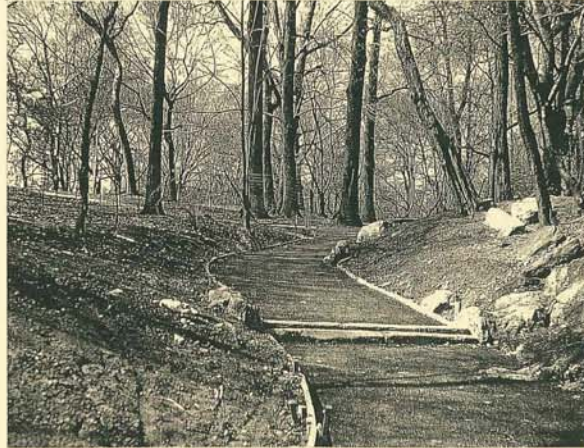
Woodland path restoration in Central Park's North Woods included drainage infrastructure and stabilization of adjacent woodland slopes which had been badly eroded and trampled. (Andropogon Associates, 1993)
