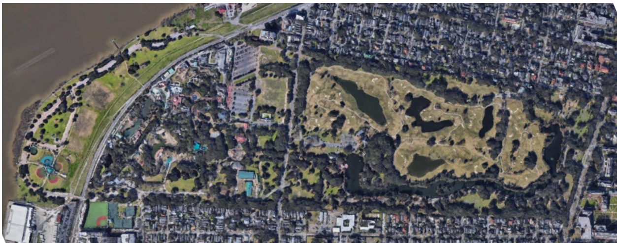
Audubon Park, Golf Course and Zoo New Orleans, Louisiana Credit: Google Earth
