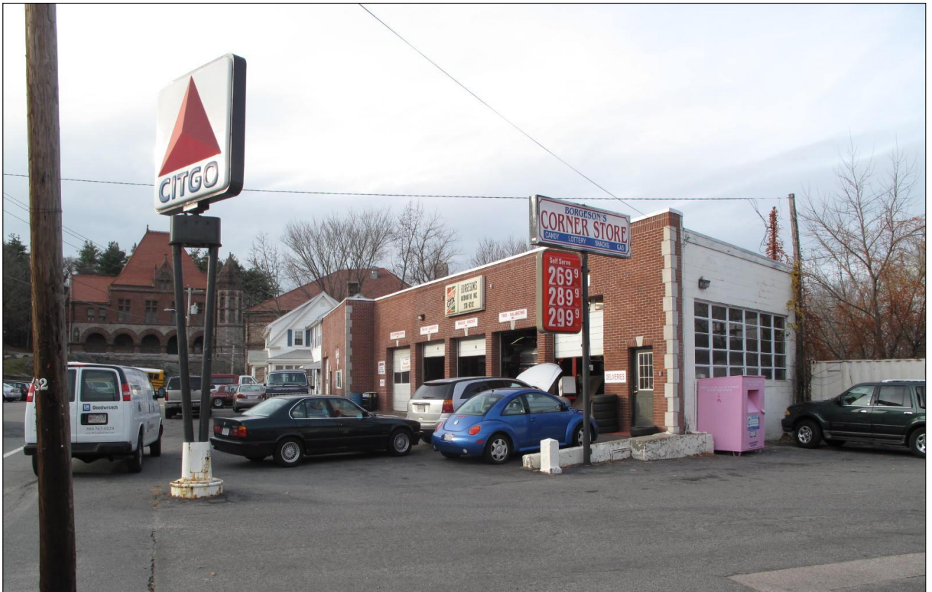
View auto repair shop from SE
