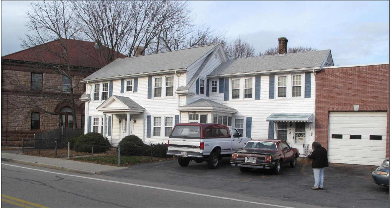
View of house from SE
