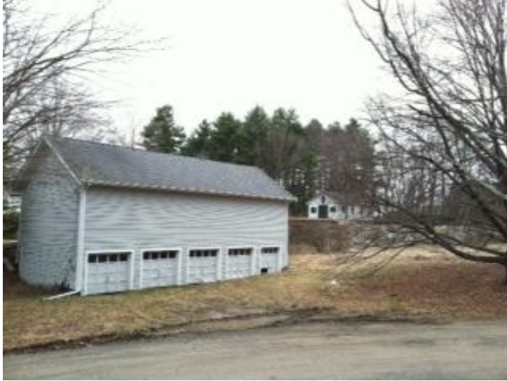
Wagon Shed foundation of Hay and Dairy Barn
