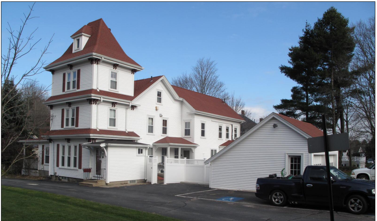
Rectory from SW
