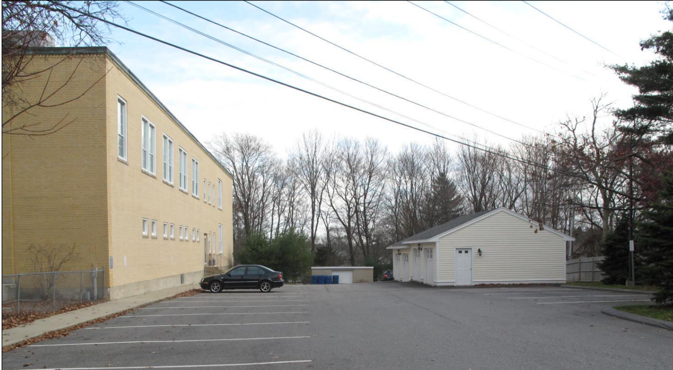
View of rear of school from W
