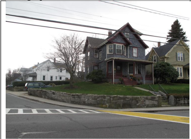
View from NE
