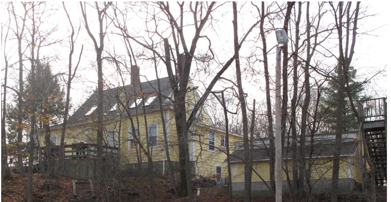
View from NE
