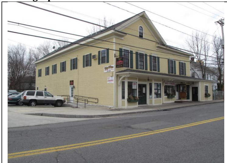
View from NE
