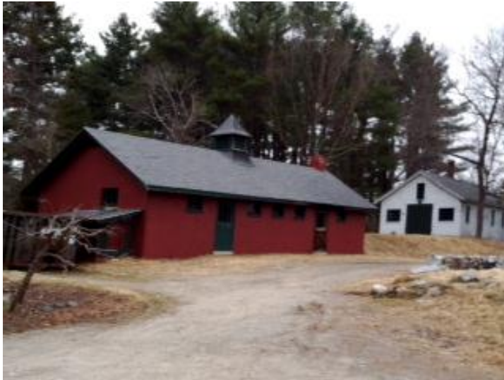
Horse Barn and Carpenter's Shop
