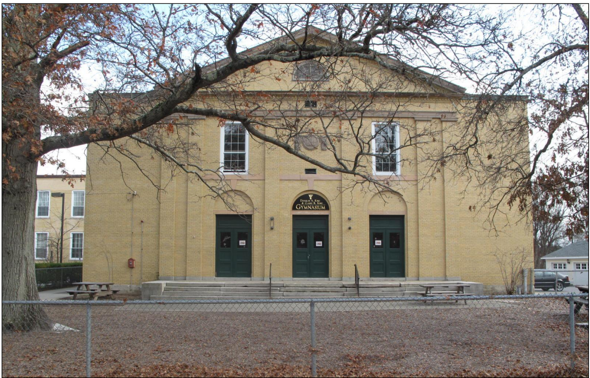
Gymnasium annex, view from W
