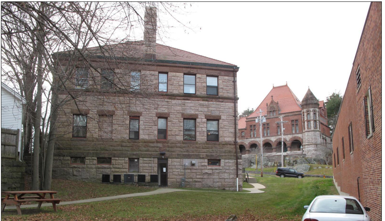
View from NE
