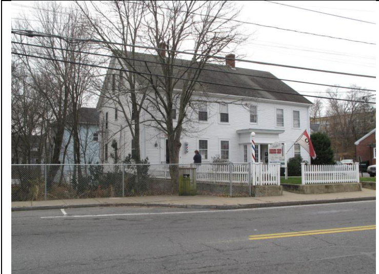
View from NE
