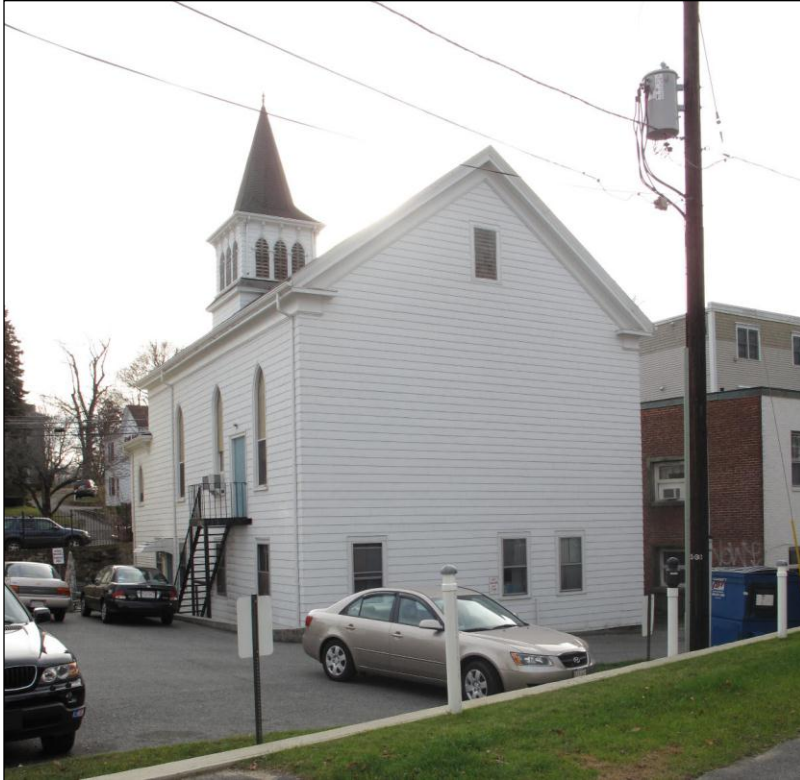
View of 140 Main from NE
