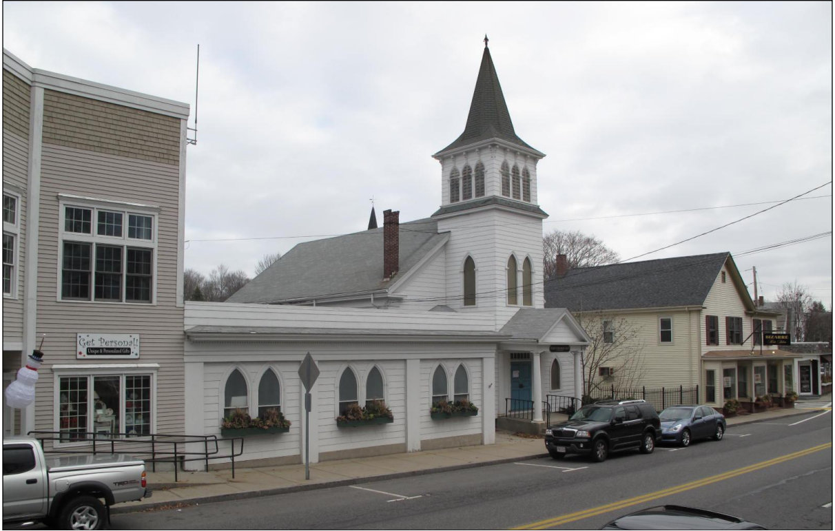
View of 140 Main from SW
