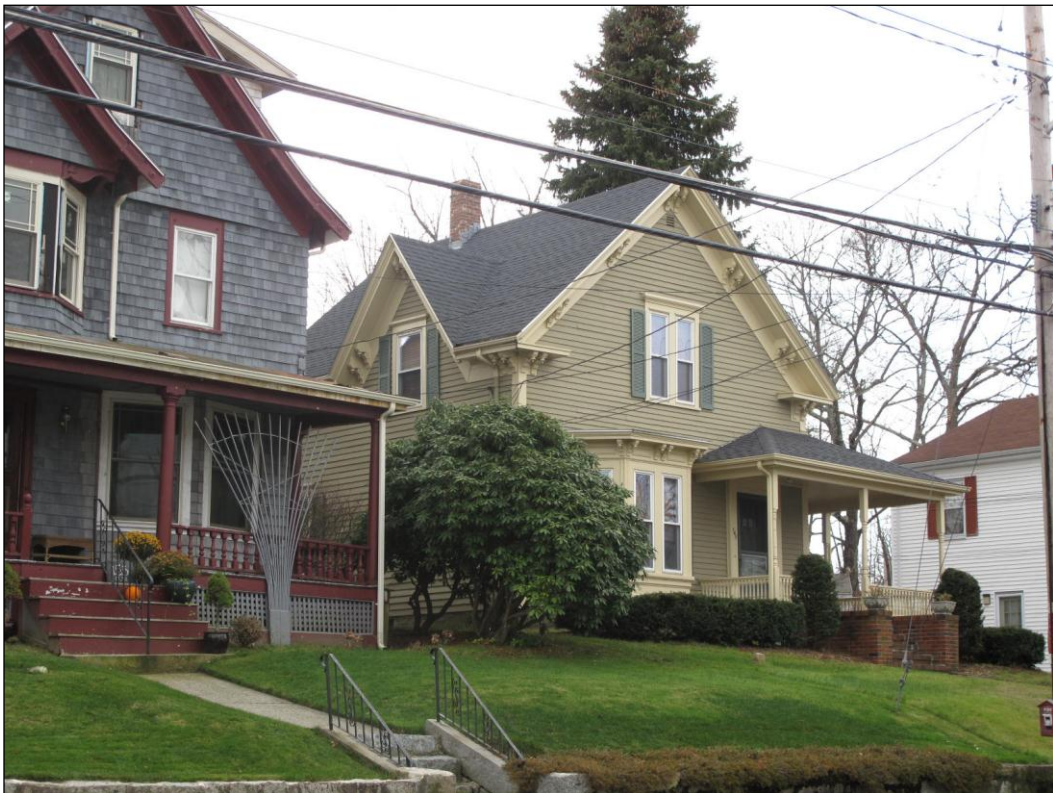
View from NE
