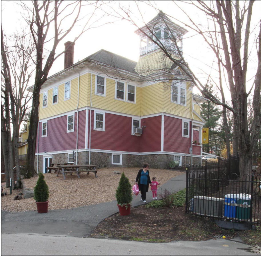
View from NE
