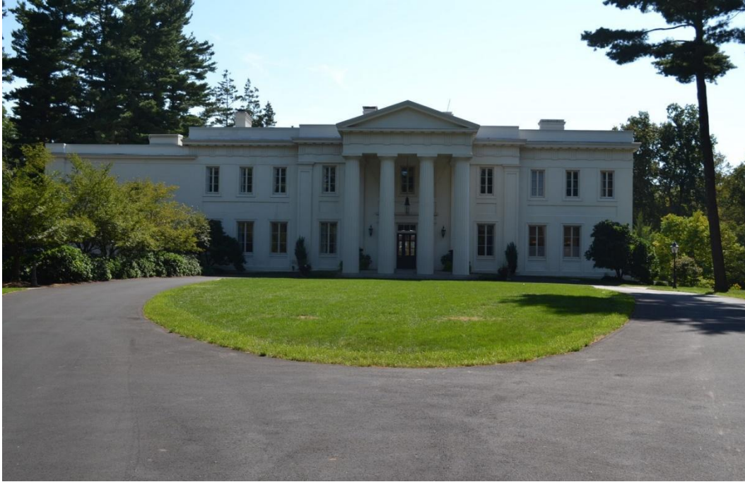
View south of the mansion from the turnaround that terminates the entrance drive.
