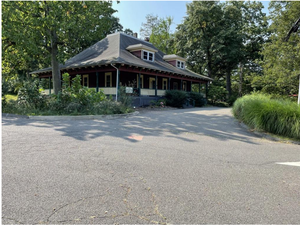
View looking east into Beardsley Zoo entrance at the historic park Casino (ca. 1884).
