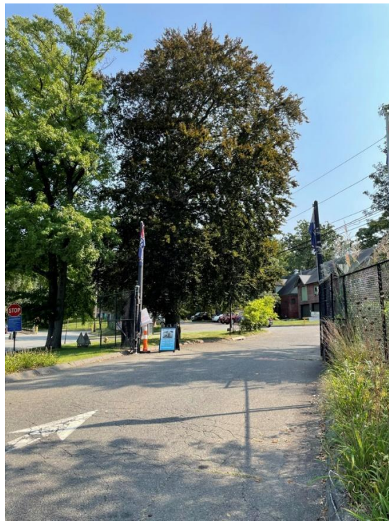
View east into Beardsley Zoo at fence. Historic brick maintenance buildings at the back of photograph (c. 1900).
