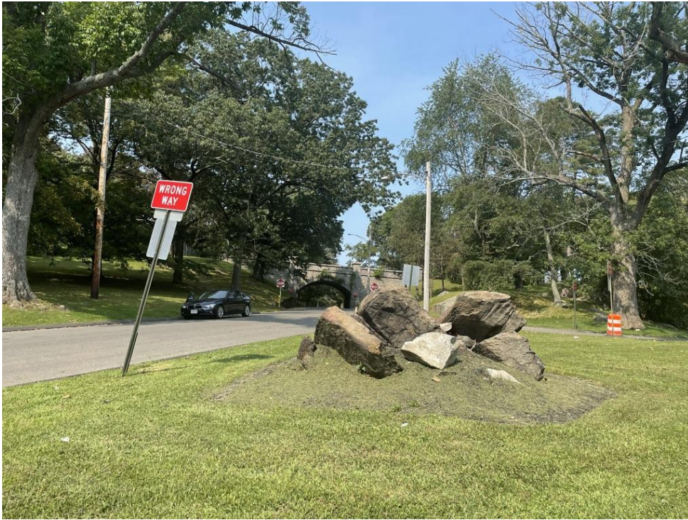
View looking west into the park exit to Rt 127/East Main Street. Note bridge that allowed a separation of traffic in the park. Upper road now abandoned.
