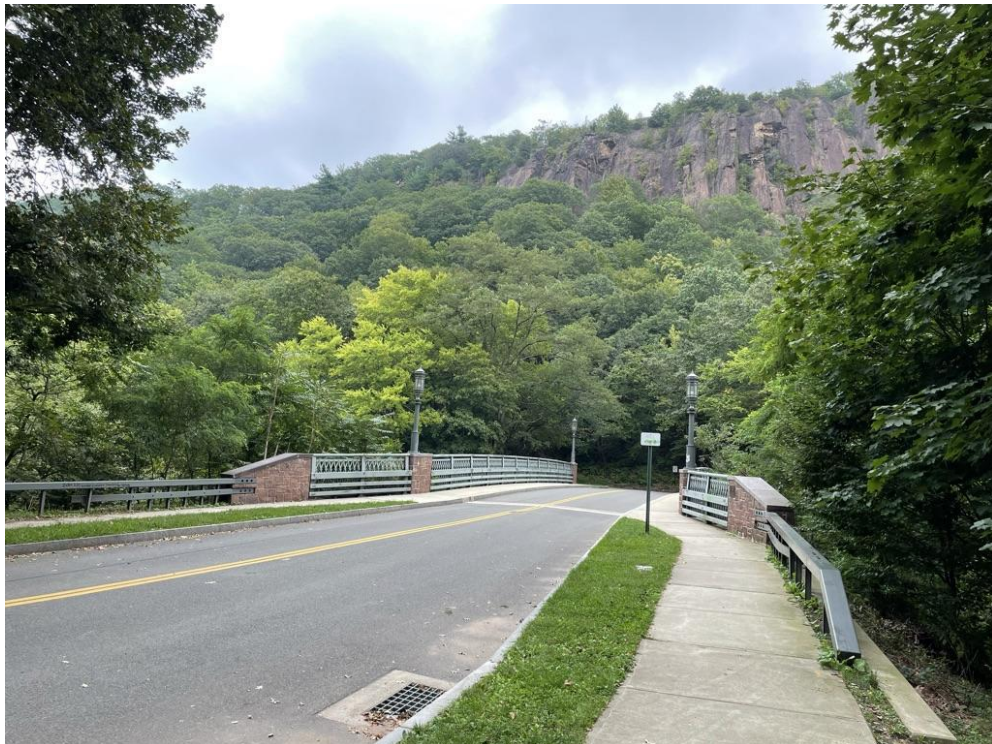
Upgraded crossing at East Rock Road at East Rock Park.
