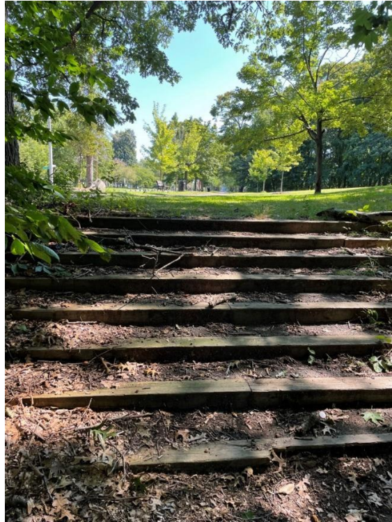
Wooden steps to accommodate pedestrians who want to circle back to upper park near Hobart Street.
