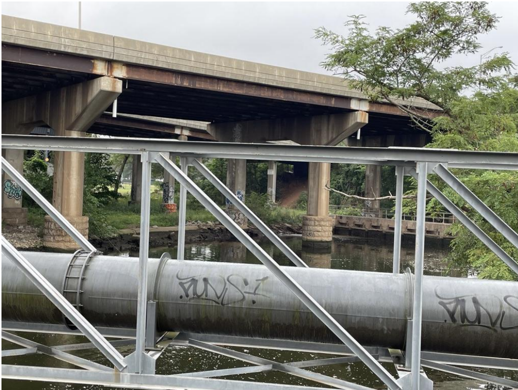
View looking north to the State Street dam that Olmsted Jr. proposed as a way to control the water of the tidal Mill River.
