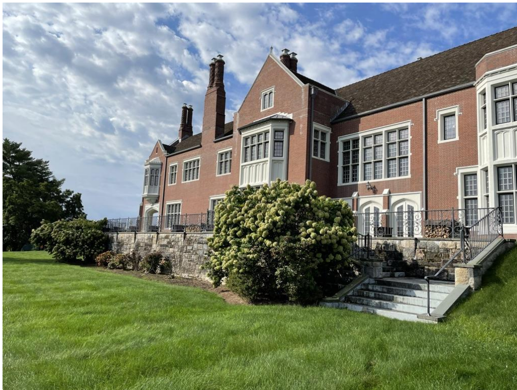
View of terrace façade of house. Stair and walls appear original. Ironwork atop walls replaced the historic stone/concrete balustrade.
