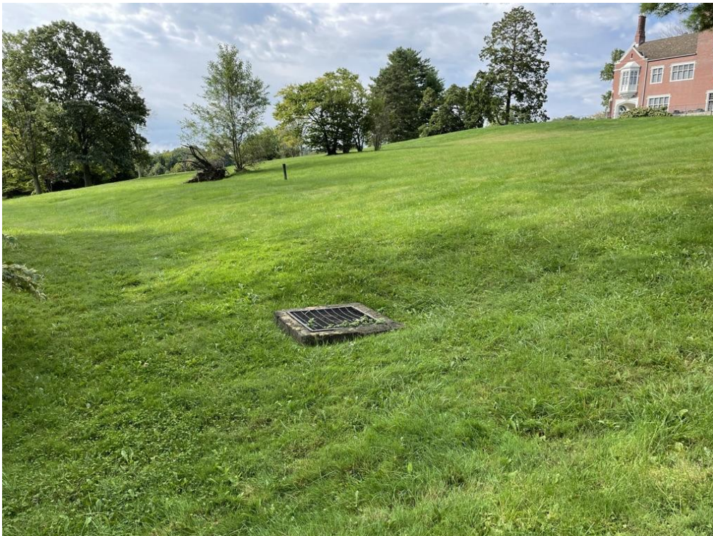
Detail view of drainage structure in lawn below house.
