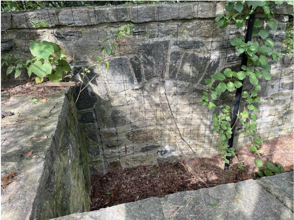
View of abandoned pedestrian access through wall at Round Hill Road.
