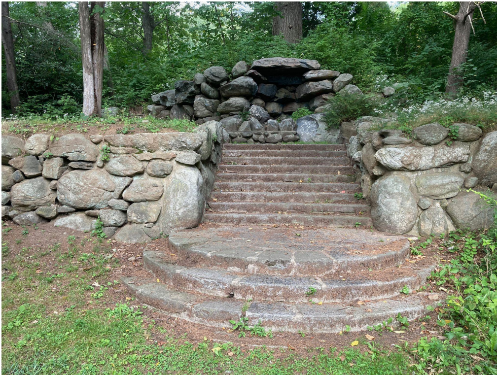
Stone grotto at top of terraces.
