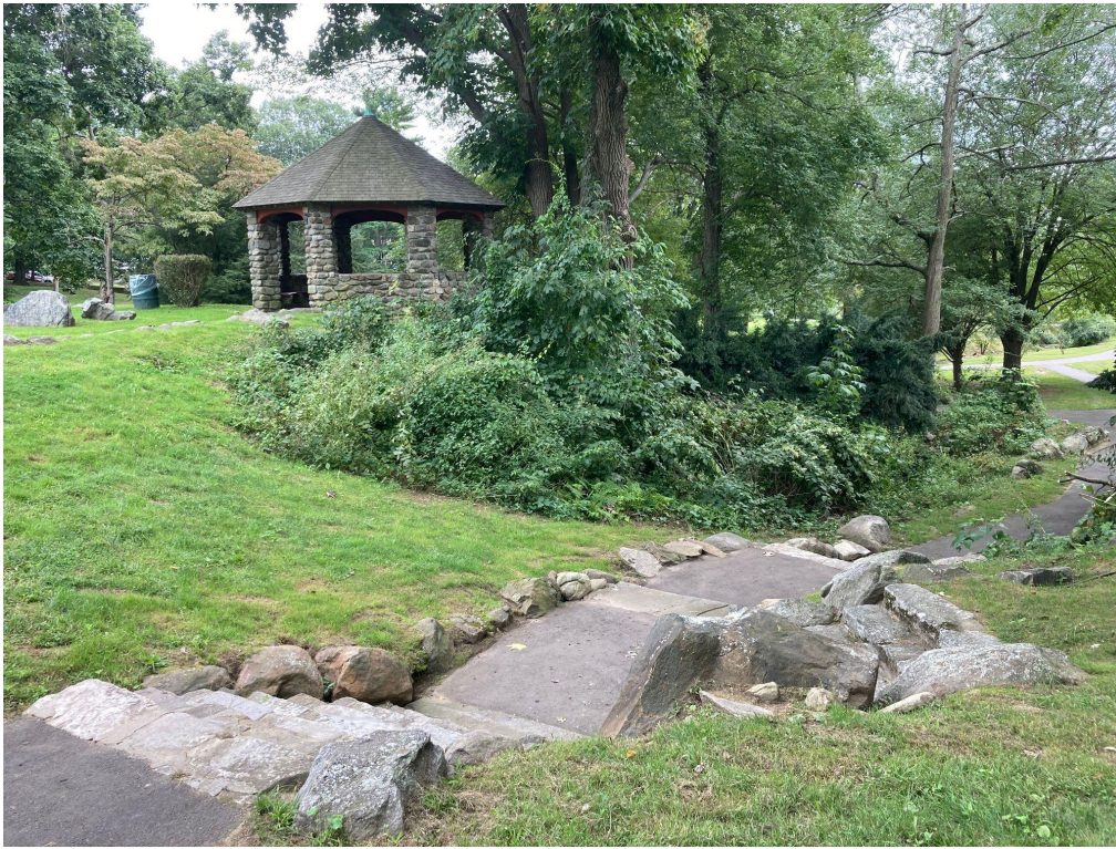
View from stairway east toward overlook pavilion.
